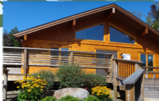
Le refuge, located on Avenue d'Anvers In Parc d'Estérel
